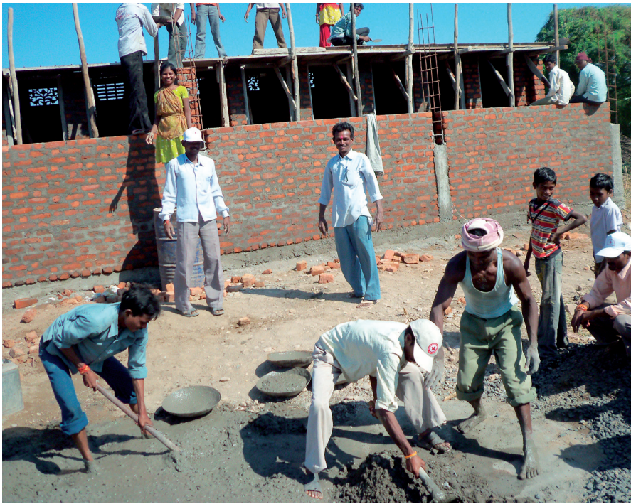
During the construction of the toilet block, the community took ownership of the project, doing much of the construction themselves.
